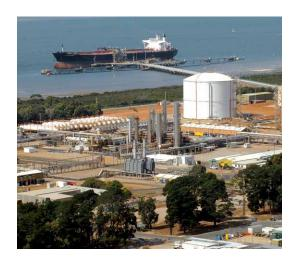
The 158 hectare site houses three gas liquids fractionation trains, 19 pressurised Liquefied Petroleum Gas (LPG - propane and butane) storage vessels, seven refrigerated atmospheric pressure LPG storage tanks, eight crude oil storage tanks, a LPG truck loading terminal and a jetty for loading LPG and crude oil onto ships. The site also has a laboratory, warehouse, workshop and administration building.
