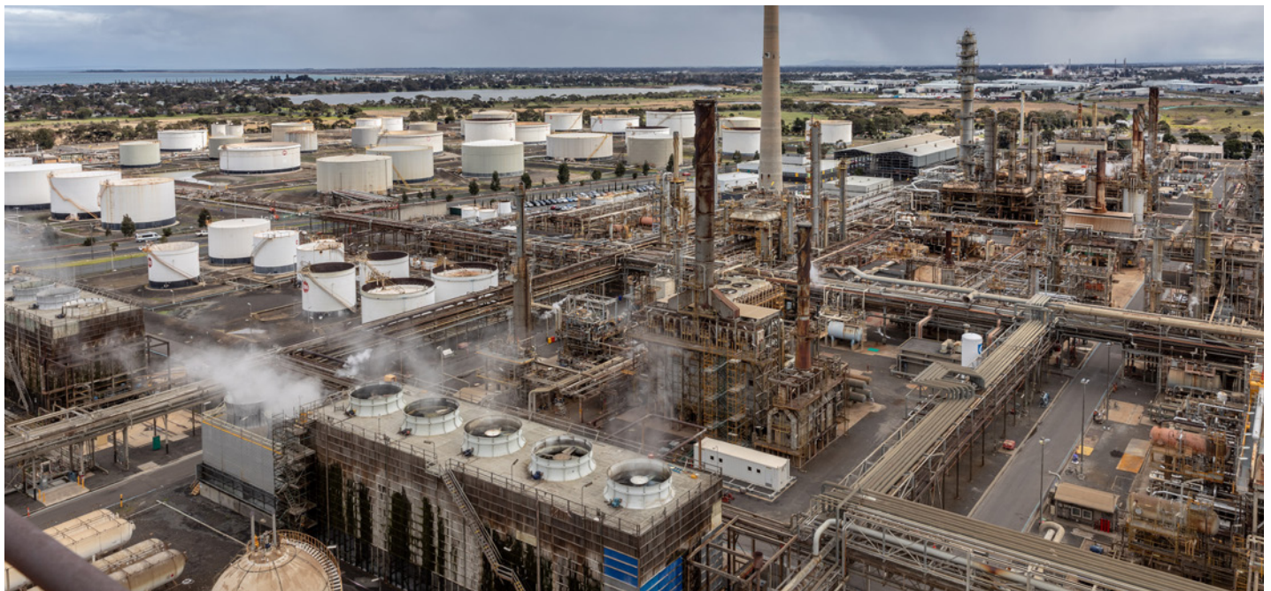
The Mobil Altona site is set to be one of Australia's key fuel storage and logistics facilities.
